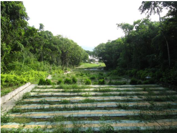
Site condition on 20/08/10
