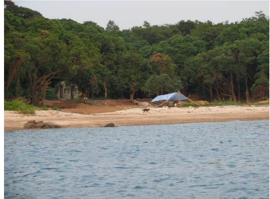
caterpilla and excavation at Shui Mong Tin
